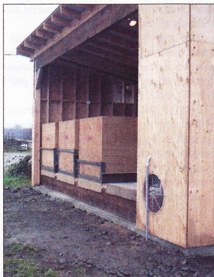
In 2011 Nash and his team constructed a new grain dryer and a structure to house it in to ensure viability of their grain seed crop over the damp winter months.
